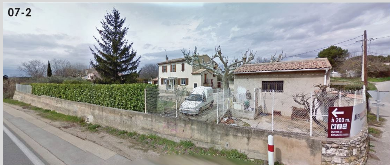
BATIMENTS A DEMOLIR
