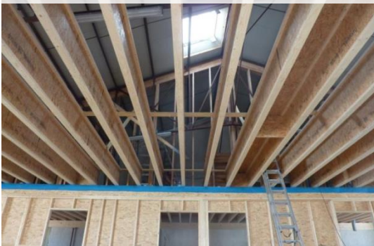
Ecole Montessori Cloisons / planchers bois
