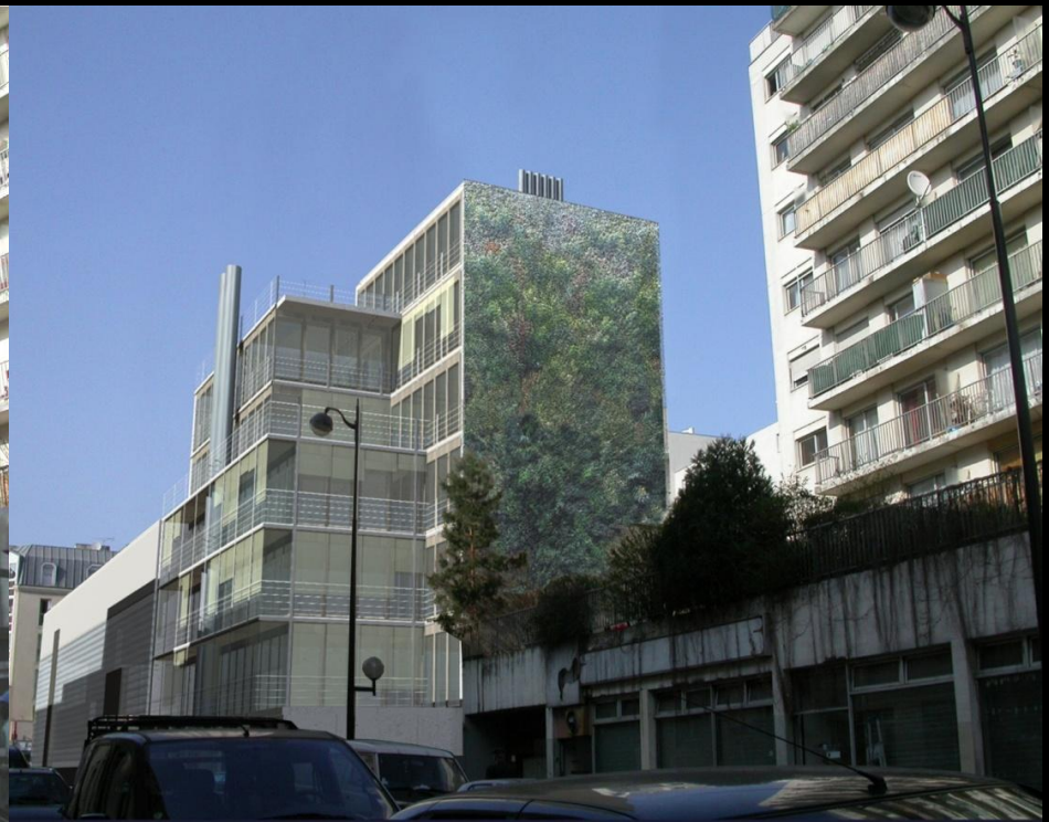
Solution construction neuve
