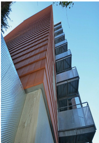
Residence Jules Ferry (ASP Architecte)
