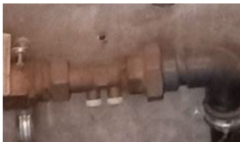
Figure 28 Clapets anti-pollution de type EA
