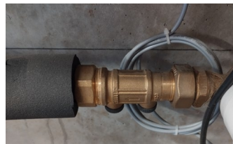
Figure 28 Clapets anti-pollution de type EA
