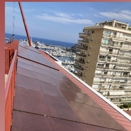
Panneaux photovoltaïque BISOL Terracotta Orange 320 Wc
