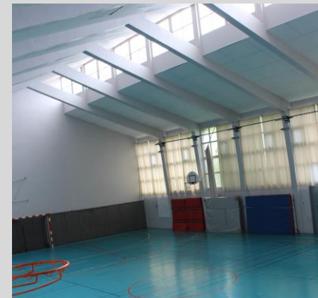
Charpente gymnase conservée
