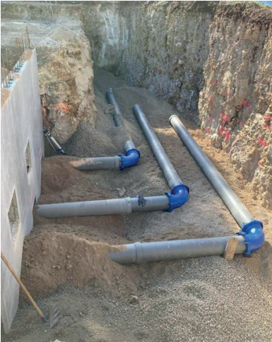
Tubes enterrés en fonte ©PamBuilding
